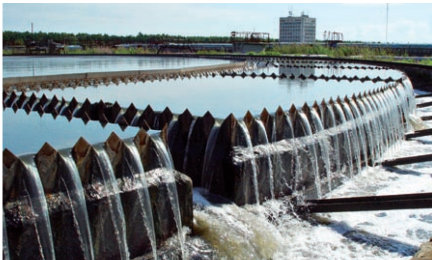
Clarifiers at St. Petersburg's southwestern wastewater treatment plant
